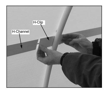
Slide the H-Channel between the panels leaving a couple inches between each piece of H-Channel. On the inside of the greenhouse, slide the H-Clip onto each end of the H-Channel pieces.
