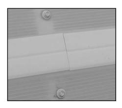
3. Slide the H-Channel pieces in so they butt together. Then put a little caulking in the joint of the two H-channels where they touch each other. In the butt joint.
